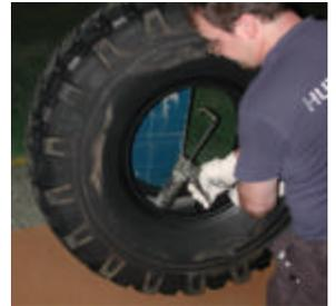
Raise the VFI with two small blocks (not included) to ease the manual VFI compression tool (Z) strap around it. Wrap the strap around the diameter of the tire and thread the end through the fastener on the compression tool, taking up as much slack as possible. (Refer to Compression Tool Strap Threading, page 15)
